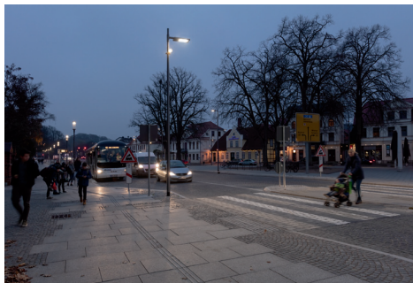
07 At the pedestrian crossing the luminaires are fitted with [P45] lenses, which WE-EF has developed especially for the illumination of pedestrian crossings and their waiting areas.
