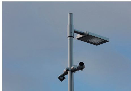
08 FLD111 projectors, which subtly illuminate the façades and accentuate selected details, are mounted on the poles of some of the VFL530 luminaires.
